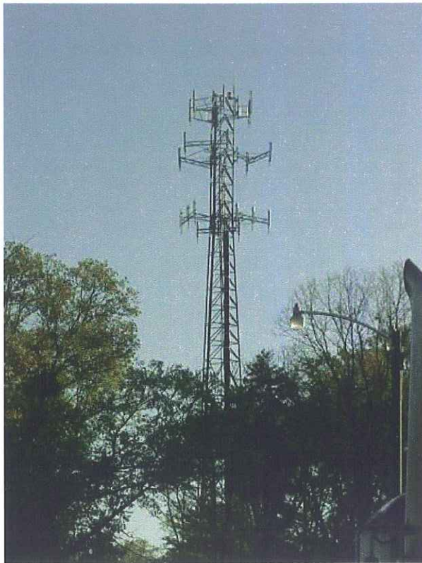
10 – Example of lattice tower – not in City.
