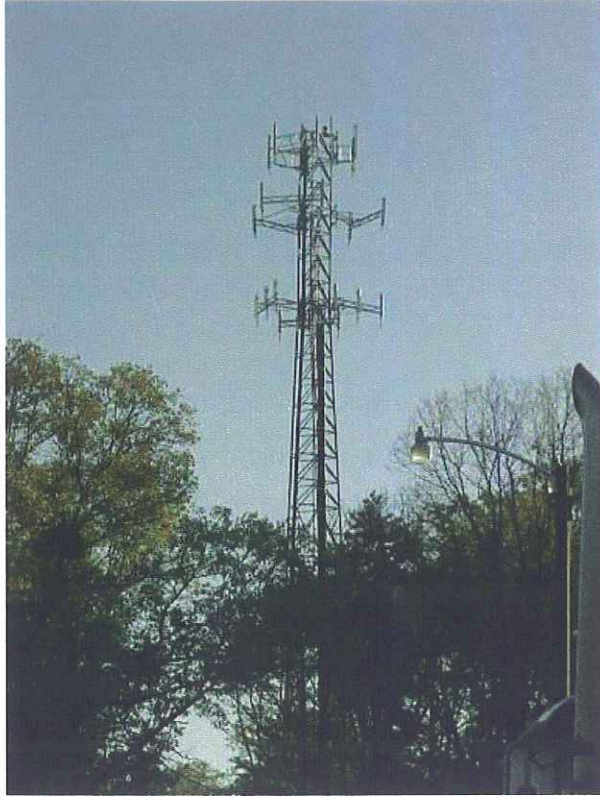
11 – Example of lattice tower – not in City.
