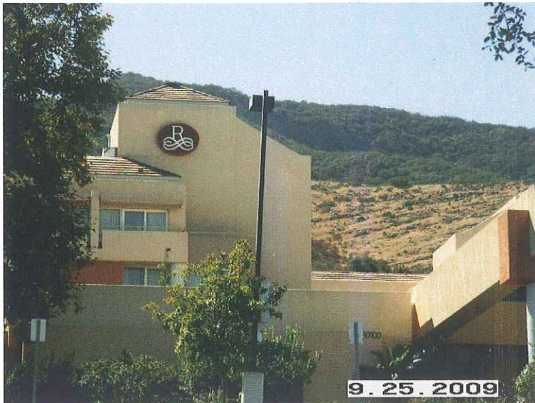
2 - Facility to right of Renaissance Hotel sign, fully enclosed in building.
