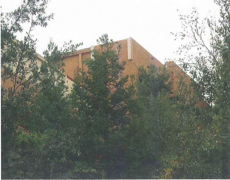
1 - White panels side mounted on Agoura Town Center Building wall.
