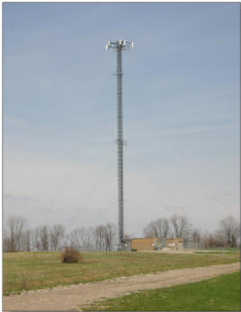
10 – Example of guyed tower – not in City.
