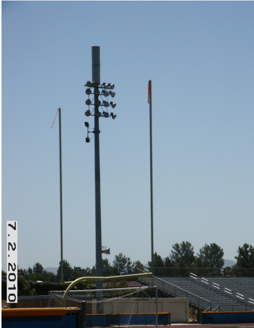
5 - Facility enclosed in cylinder on top of stadium lighting at Agoura High School.
