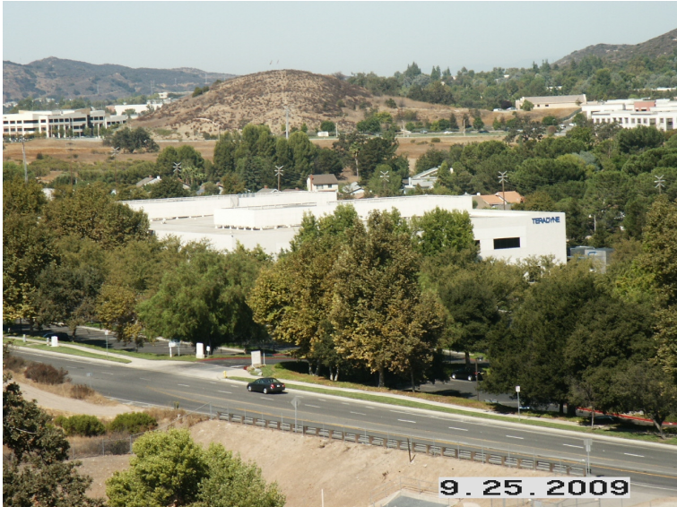
3 – Equipment screened by roof parapet wall on former Teradyne building.
