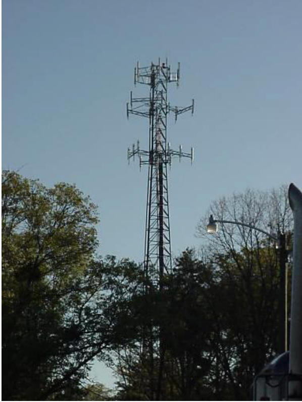
11 – Example of lattice tower – not in City.
