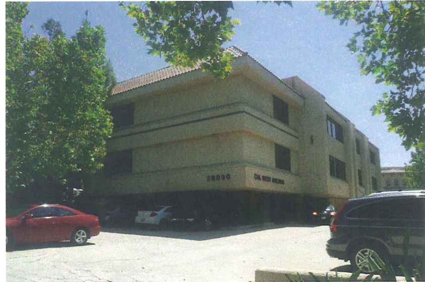
NORTHWEST CORNER VIEW OF THE BUILDING
