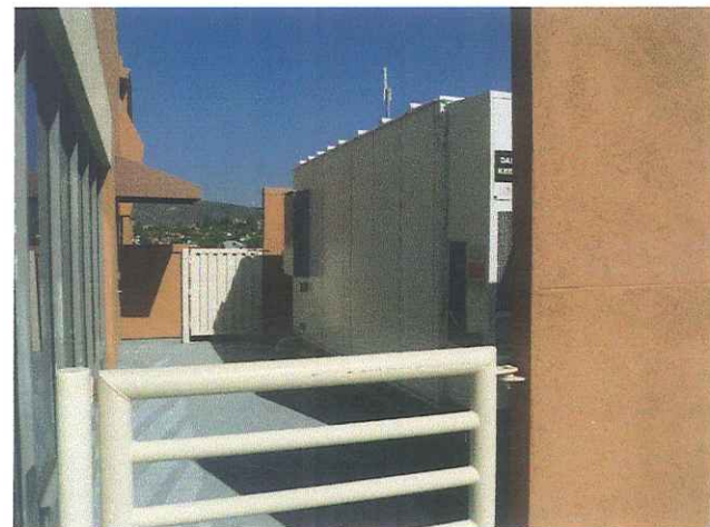
ROOF TOP VIEW OF EQUIPMENT SHELTER
