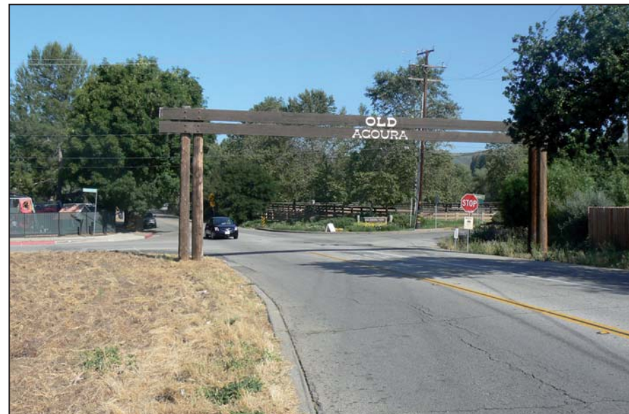
Photo 4 - View of entrance to Old Agoura looking west.
