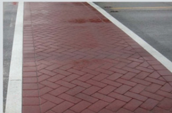
Crosswalk with integral color, stamped asphalt
