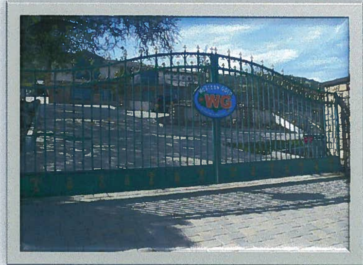
Luithly Office Building Conversion
