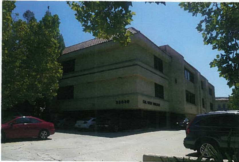
NORTHWEST CORNER VIEW OF THE BUILDING
