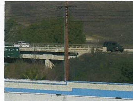
Palo Comado Interchange Bridge
