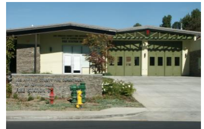
Fire and emergency services in the City are provided by the Los Angeles County Fire Department
