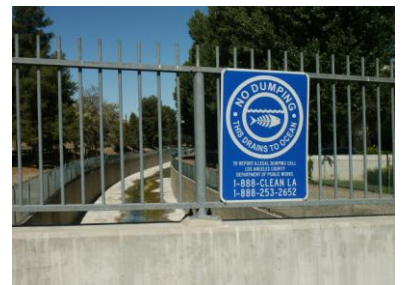
Flood control and storm water facilities
