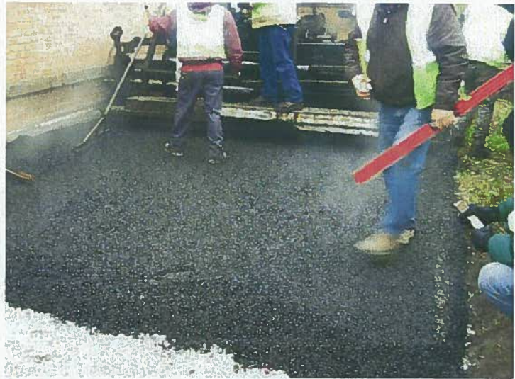
Figure 9: Permeable Asphalt Installation Using Ground Tire Rubber.
