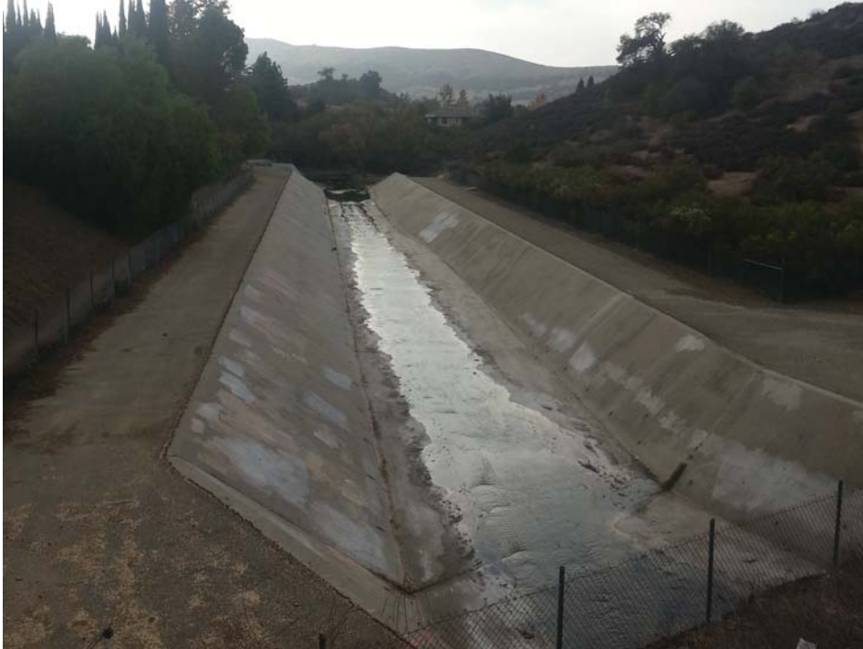
Photo 1: View of concrete-lined creek channel, facing southeast.
