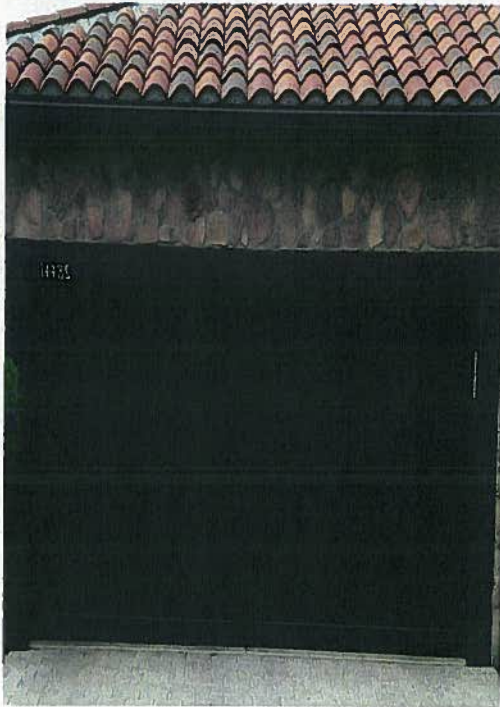
Garage Door, Stone & Roof
