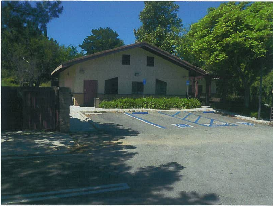
WEST VIEW – BUILDING ENTRANCE
