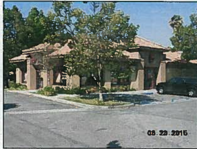
2 NEC BLD'G FROM PARKING LOT
