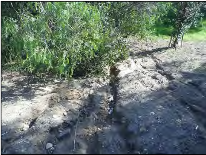
Photo 3C – Erosional features on the south facing side-slope of US 101 are shown. Runoff from this slope drains to a topographically low area along the northern property boundary, resulting in mesic but not wetland conditions.
