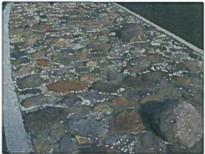
STONE COBBLES (MEDIANS) - RIVER ROCK COBBLES, ROUNDED 3" TO 6" SIZE, COLOR: YOSEMITE MIX
