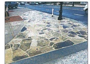
FLAGSTONE PAVERS - 1-1/2 TO 2" THICK MAX, SIZES 12" TO 18" DIAMETER, COLORS: MATCH EXISTING
