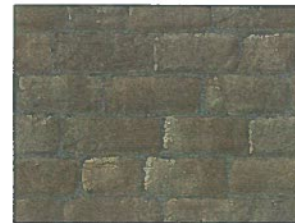
KEY INTERSECTION PAVERS (BAND) - BELGARD PAVERS OLD WORLD PAVER, COLOR: BLENDED MONTECITO
