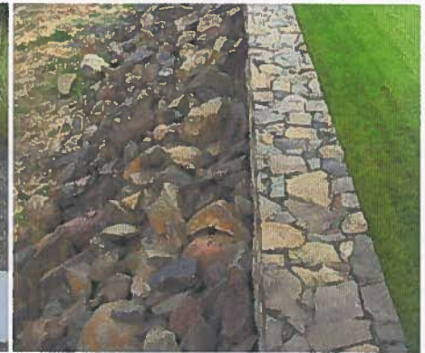
3. Stone Wall with Cobble Blanket
