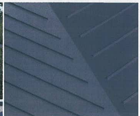
12. Standing Seam Roof
