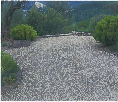
1. Chip Seal Paving
