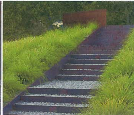
5. Gravel Stair with Steel Edging
