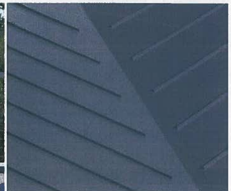
12. Standing Seam Roof
