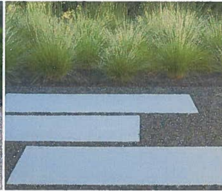
2. Concrete Pavers in Gravel
