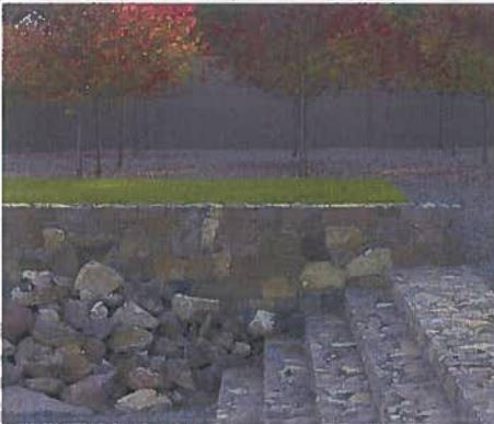
4. Stone Wall and Stair
