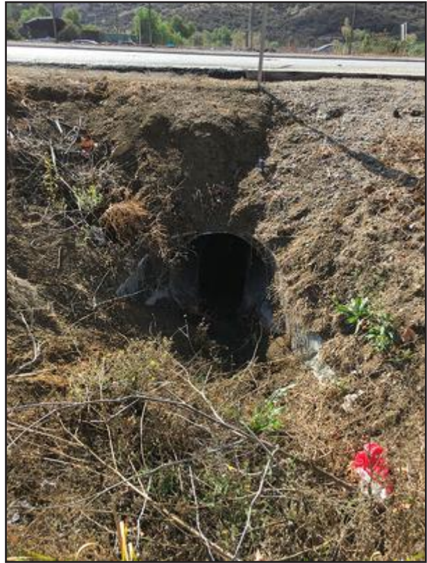
Photo 2 – View to the south of the culvert under Canwood Street at the southern terminus of the ephemeral drainage. The drainage is supplemented by irrigation runoff from the adjacent medical plaza.
