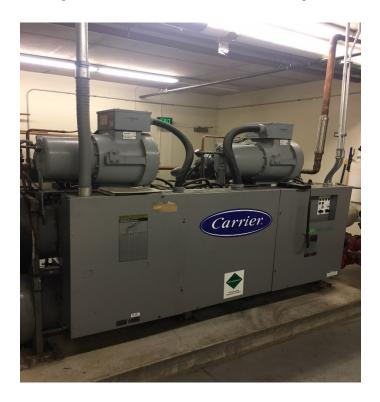
HVAC Chiller Compressor Replacement/Installation
