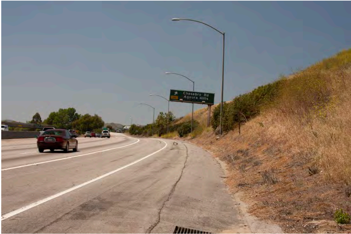
Figure 2.3: VL1 – Existing Condition NB Off Ramp
