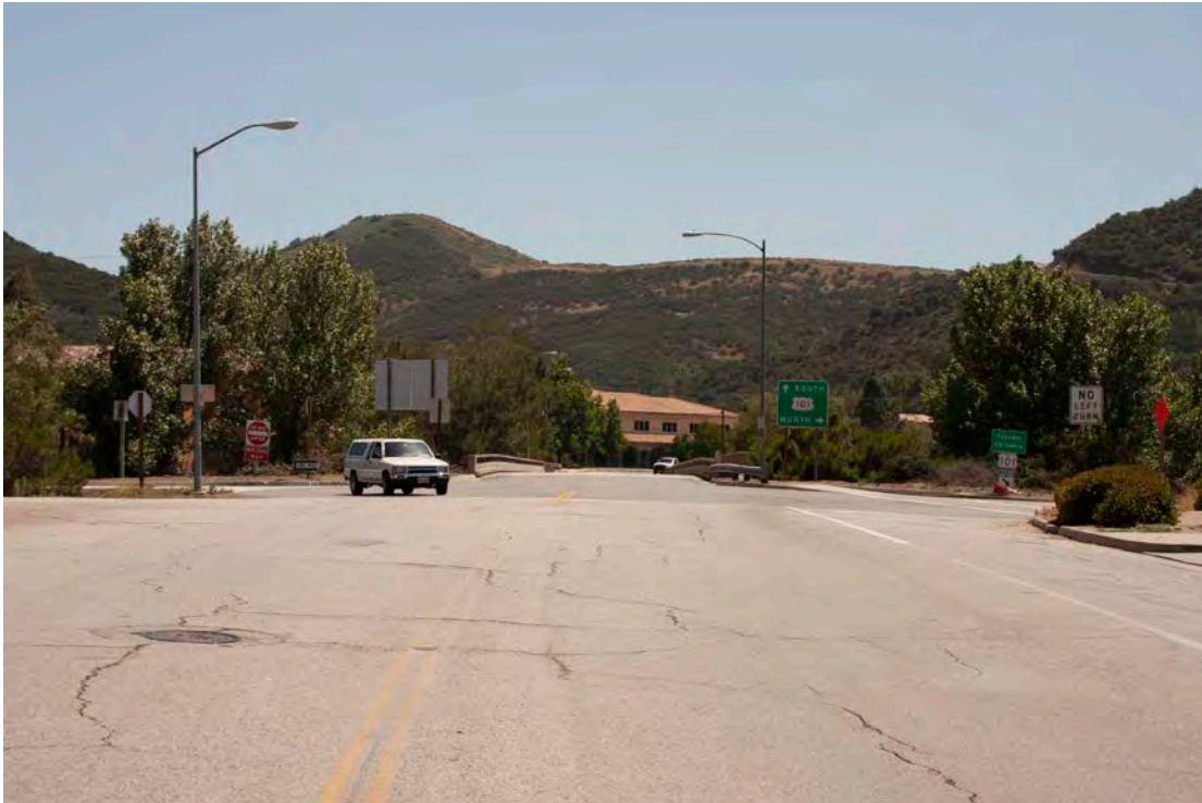
Figure 2.5: VL2 – Existing Condition Looking South at the Overcrossing
