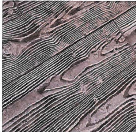
(2) Board formed concrete boardwalk pavers
