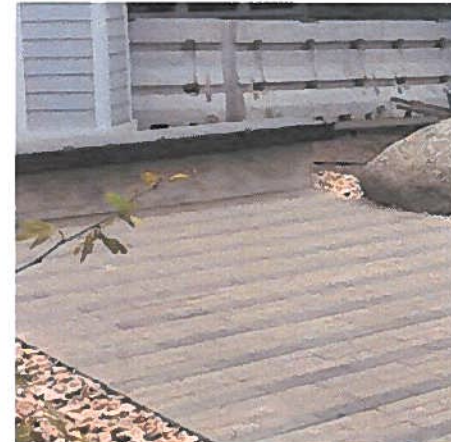
Seatwalls w/ board formed concrete face
