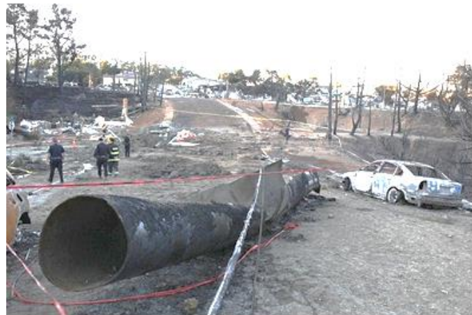
Figure 67: San Bruno Pipeline Explosion
