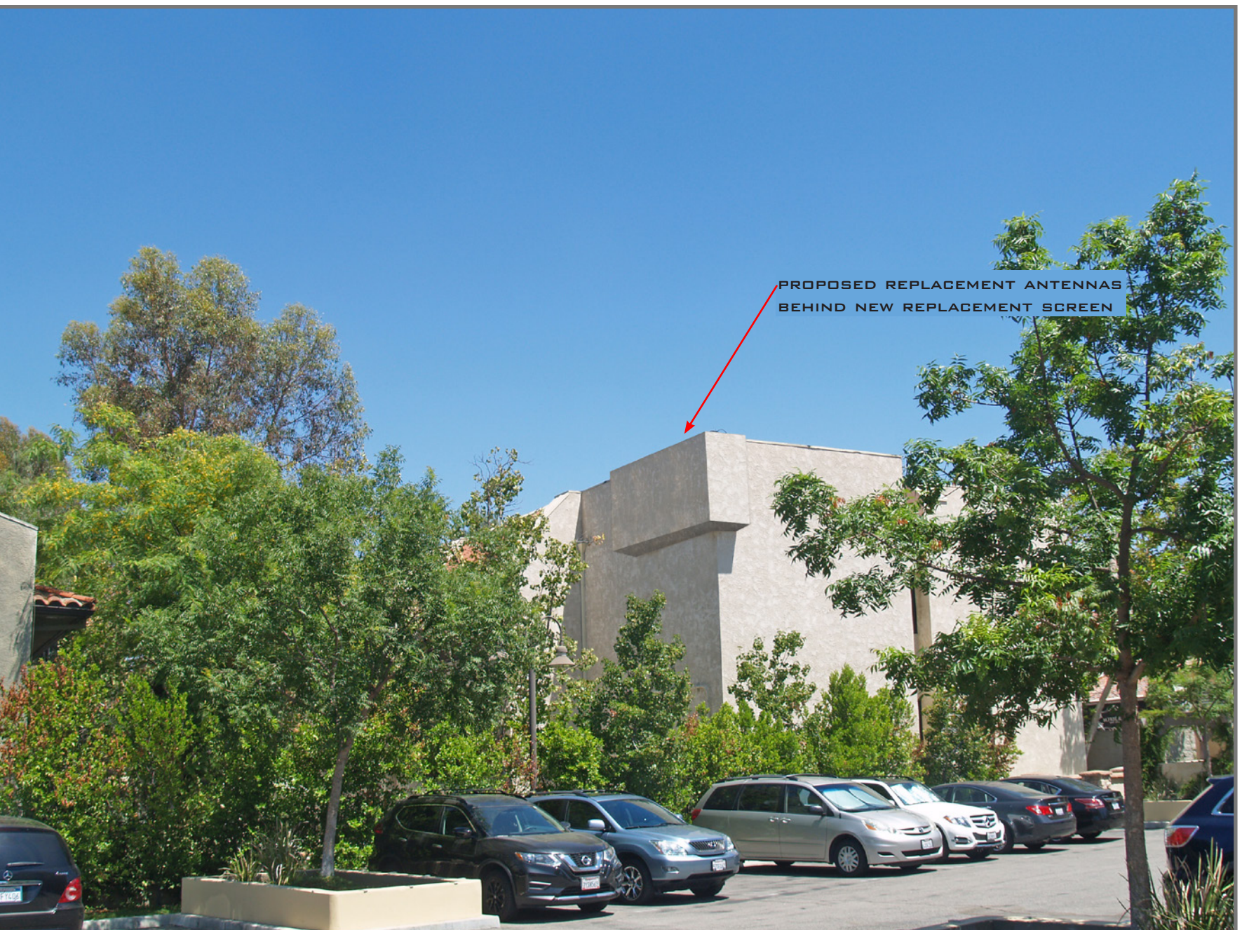
LOOKING NORTHEAST FROM ADJACENT PARKING LOT
