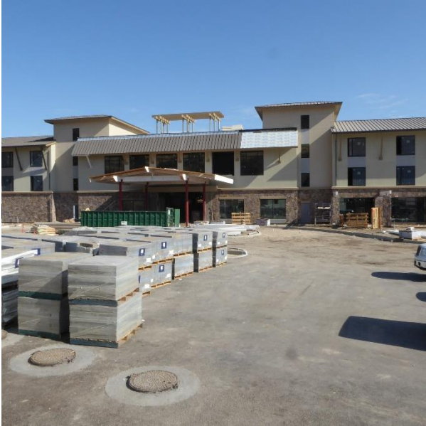
Front Elevation of the Hotel
