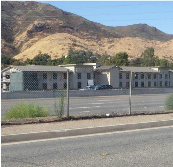
Rear Elevation of the Hotel
