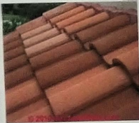
#1: Concrete Roofing Tiles - Eagle Roofing 3125 Capistrano
