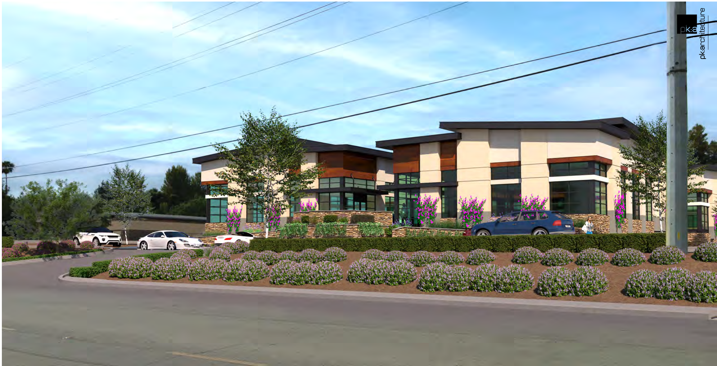
View from Canwood Street Looking North
