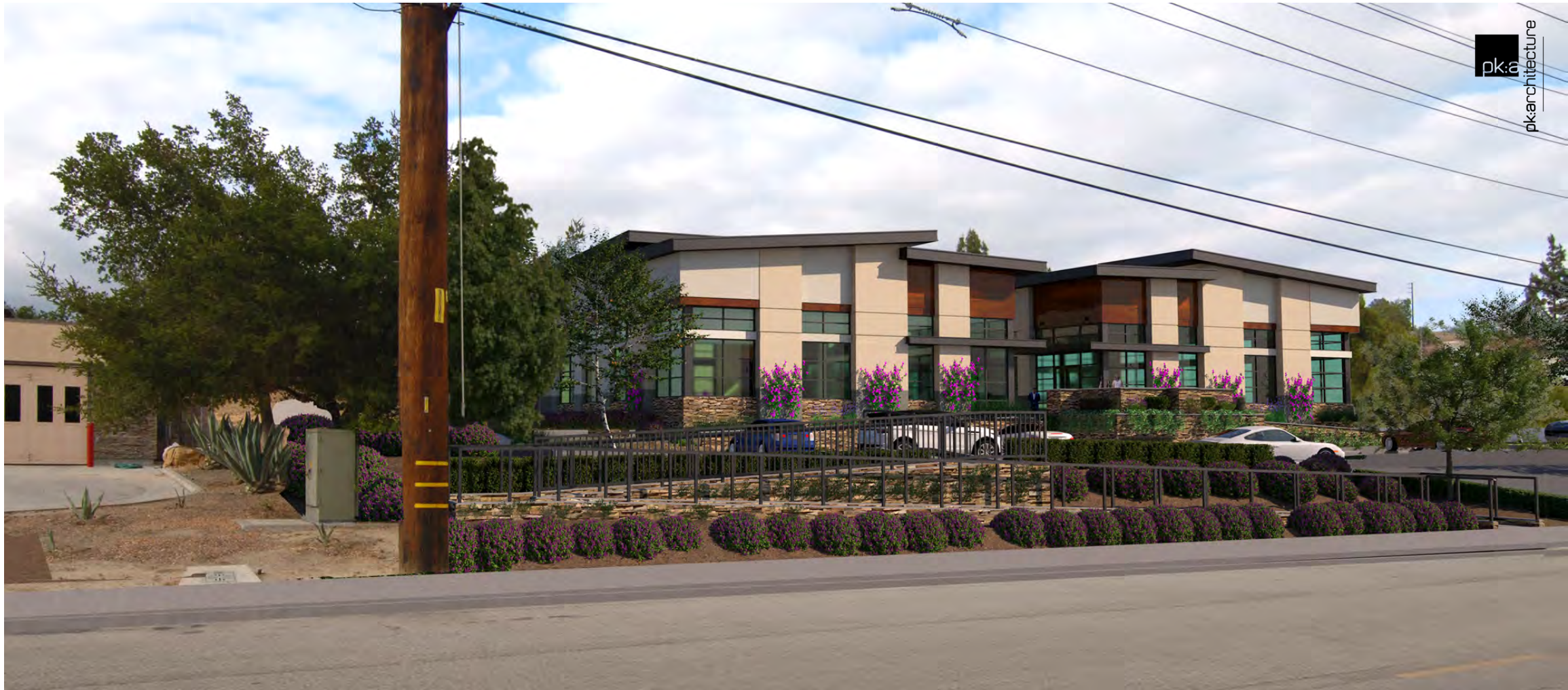
View from Canwood Street Looking North
