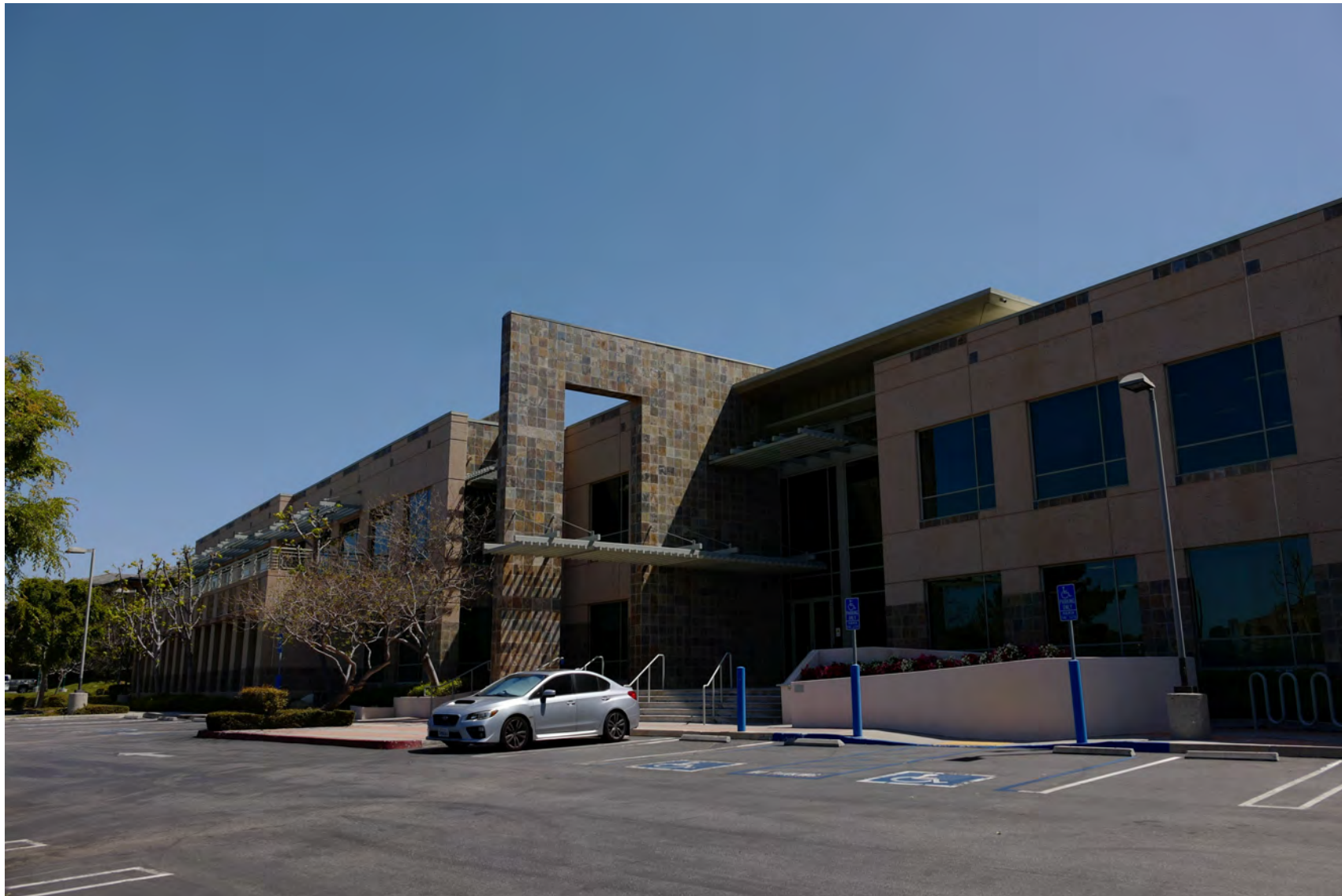
30301 Agoura Road, Agoura Hills City of Agoura Hills Compatible Architectural Design Example
