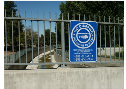
Flood control and storm water facilities
