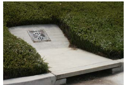
Stormwater drain on Agoura Road and Laura La Plante Drive
