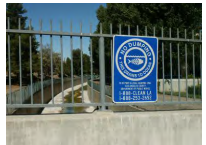
Flood control and storm water facilities
