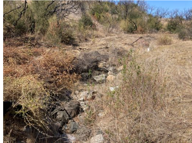
Photo 4. View of the potentially jurisdictional aquatic resource/drainage located in the southern segment of the Roadside portion of the survey area, facing southwest (34.144170, -118.767242).
