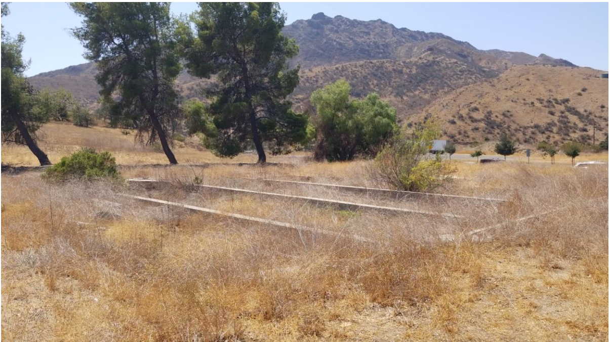
Photo 4: Modern Building Footings (View SW)
