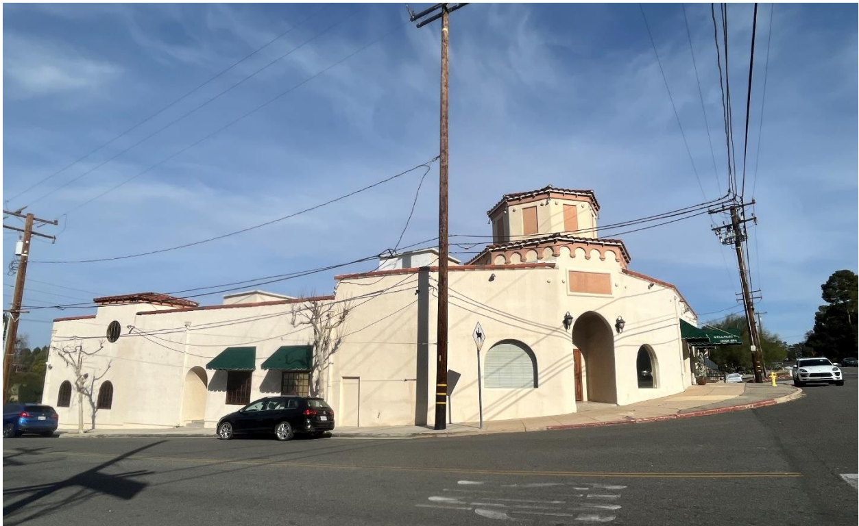
Figure 3 Old Post Office, as Observed During the Survey
