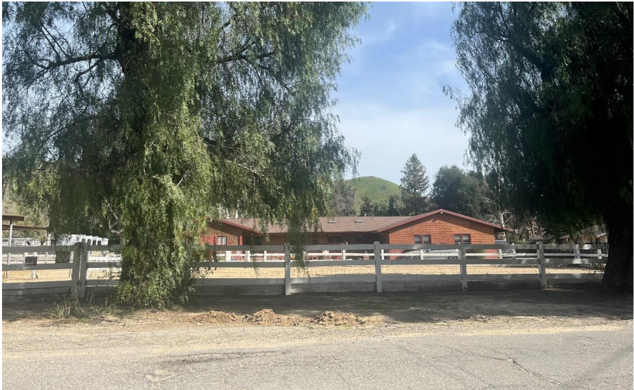
Figure 7 Representative Photo: Residential Property Characteristic of Old Agoura
