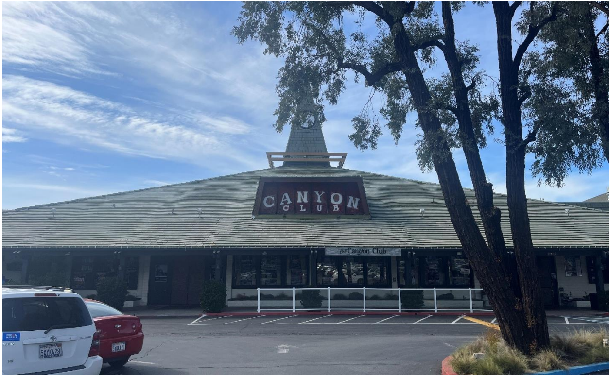
Figure 10 The Canyon Club, as Observed During the Survey
