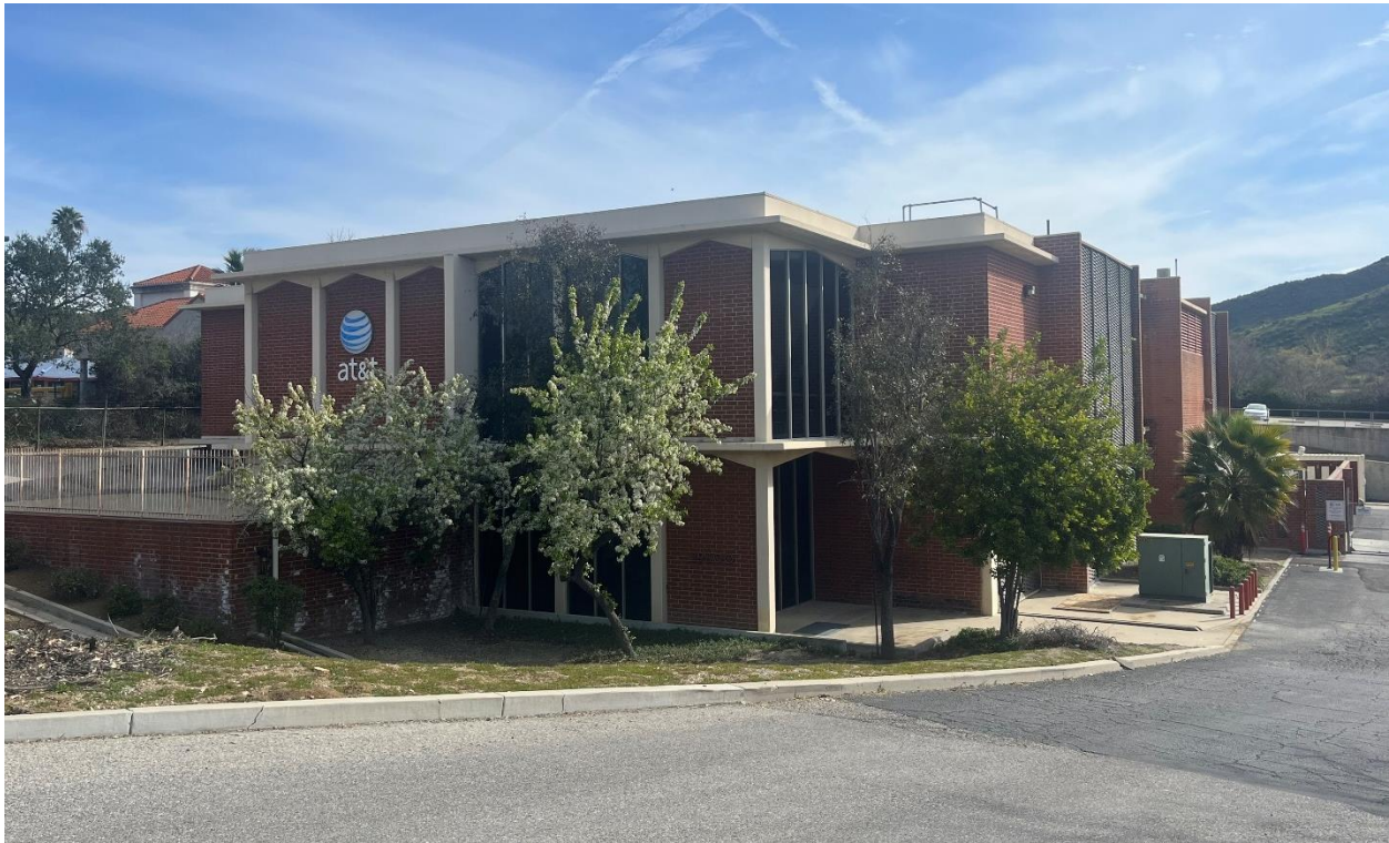
Figure 12 AT & T Building on Roadside Drive, west of Kanan Road as Observed During the Survey
