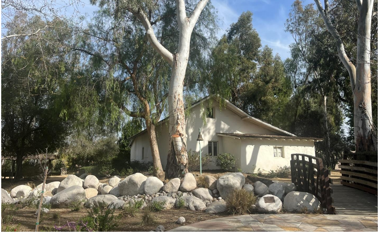
Figure 2 Reyes Adobe, as Observed During the Survey
