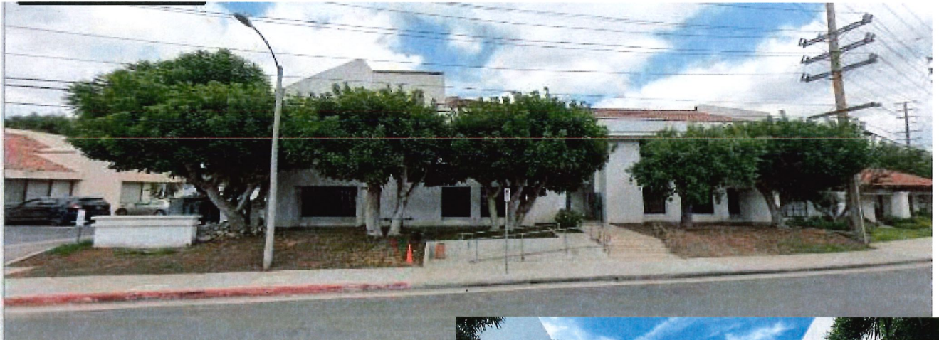
Front Elevation of the Building
