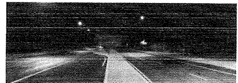
High pressure sodium led to the right was replaced with 3,000K adaptive LED. Photo shows the LED fixture by Jim's Barnhouse.
