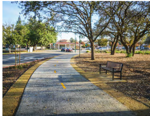
Existing trees are maintained to provide shade and respite along bike path.
