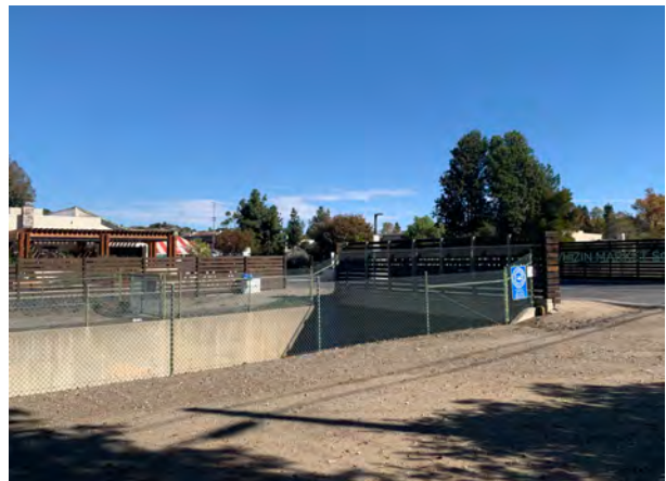
Concrete channel along Agoura Road at the Whizin Market Square.
