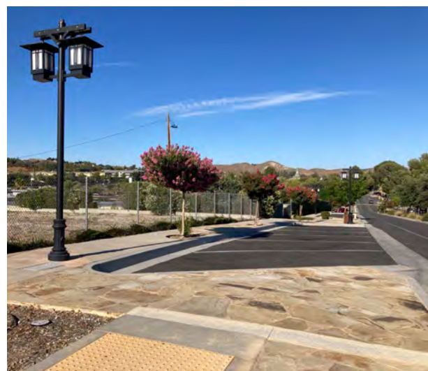
Flagstone Pavers with integral color concrete sidewalk
