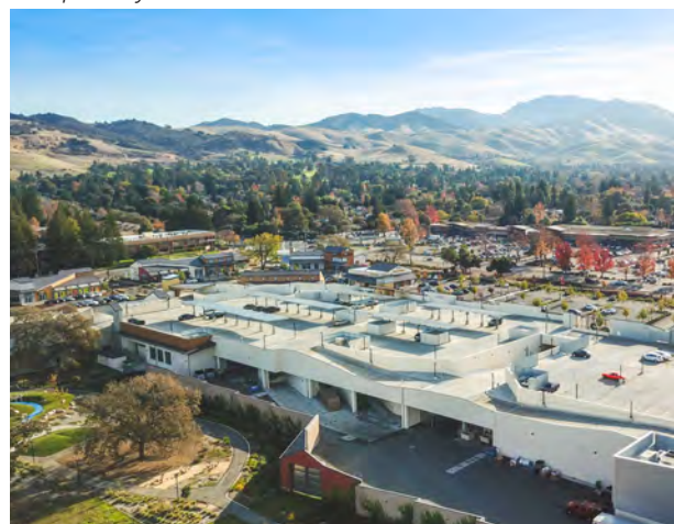
Roof mounted equipment on parking structure are screened from public view.
