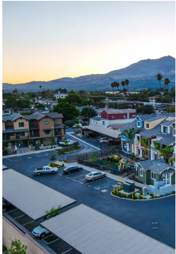
Covered parking incorporated into the project.
