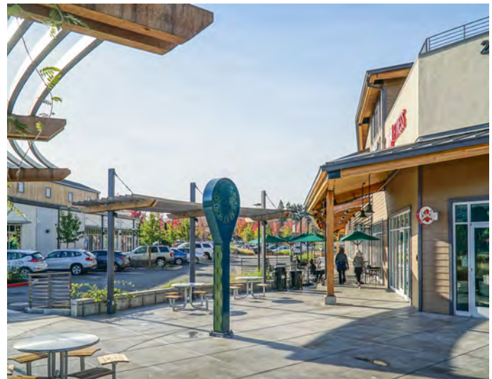
Buildings along internal streets provide ground floor transparency and amenities within setbacks.
