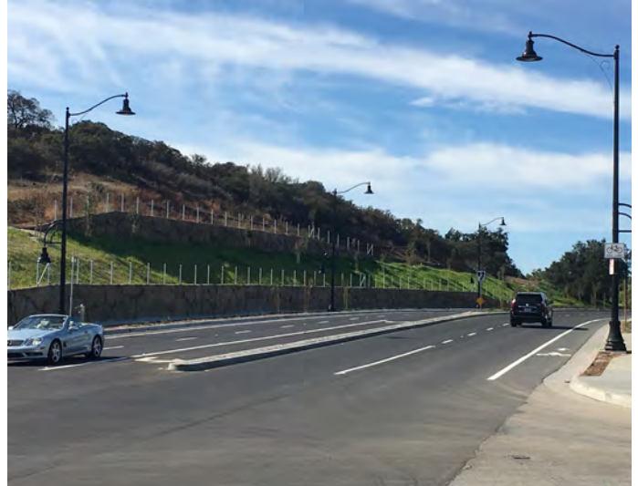
Retaining walls in Agoura Hills provide an example of textured materials that simulate rocks.
