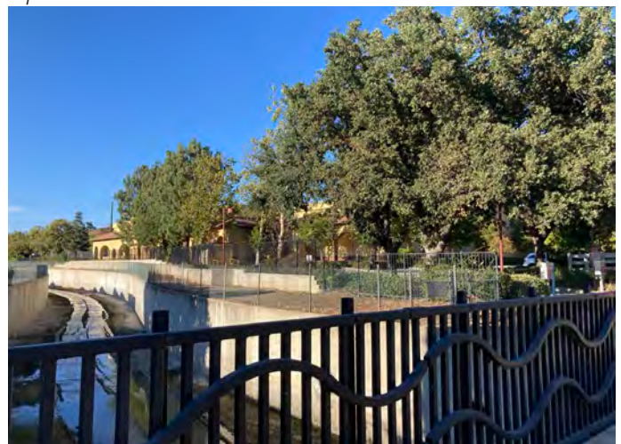
View looking north along the Medea Creek channel.
