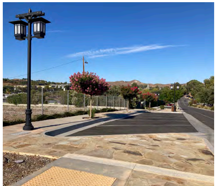
Flagstone Pavers with integral color concrete sidewalk
