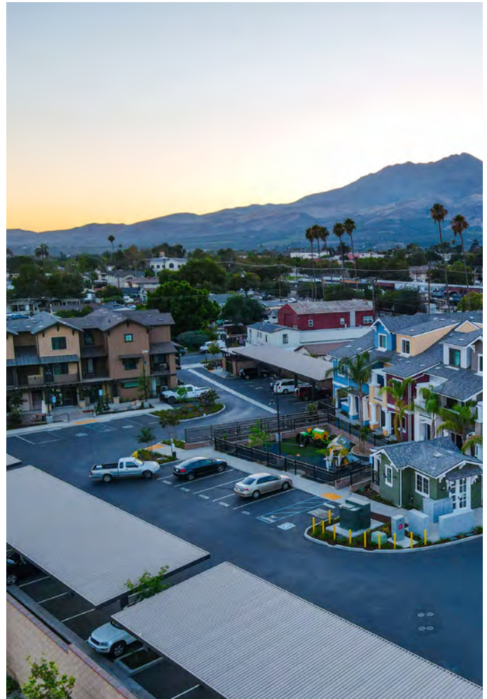
Covered parking incorporated into the project.
