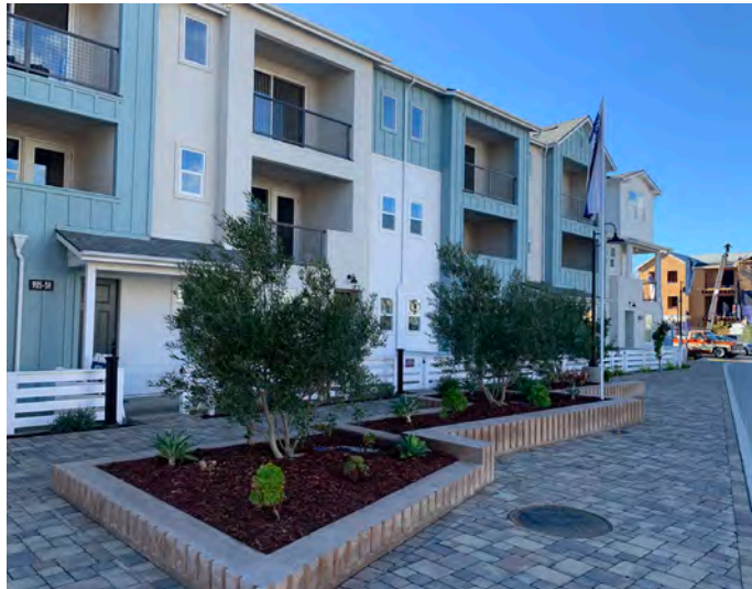
Architectural elements, recessed balconies, and changes in materials contribute to facade articulation.
