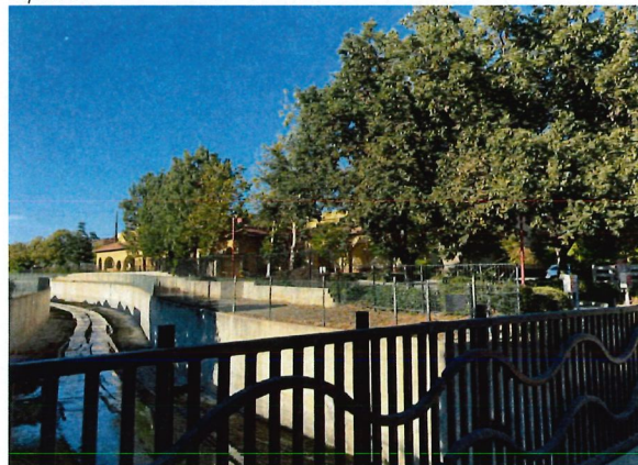
View looking north along the Medea Creek channel.
