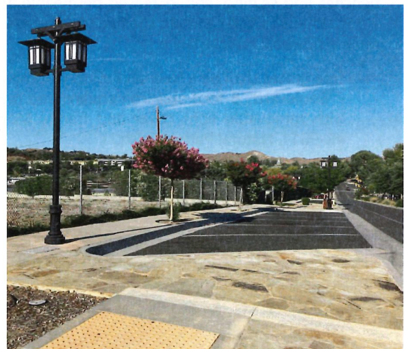
Flagstone Pavers with integral color concrete sidewalk
