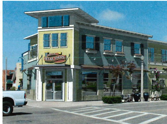
Primary building entry is enhanced with building form and articulation.
