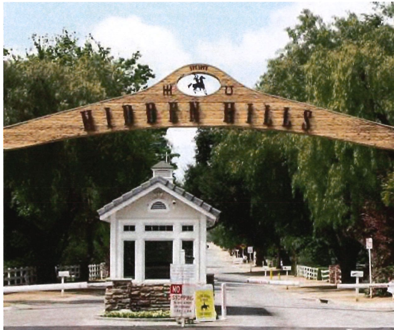
Figure 34: City of Hidden Hills Entrance Gate
