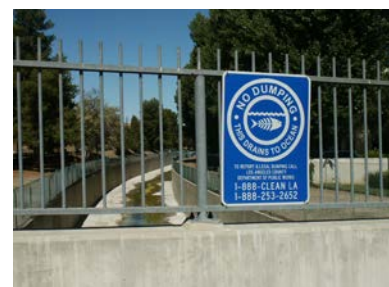
Flood control and storm water facilities
