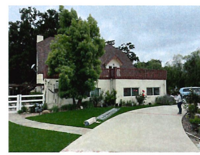
3 VIEW OF EXISTING FRONT SFD FROM DRIVEWAY
