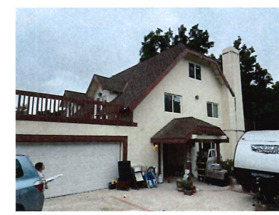
4 VIEW OF EXISTING COVERED ENTRY PORCH
