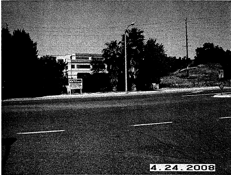
Looking North at the Project Site
