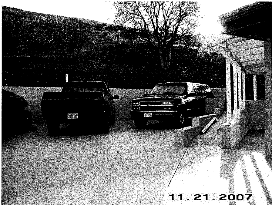
Rear of the Building
