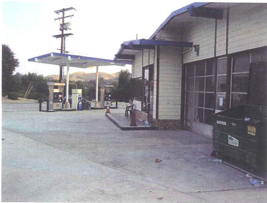
#4 Looking northwest – the maintenance shop has moved to another location.
