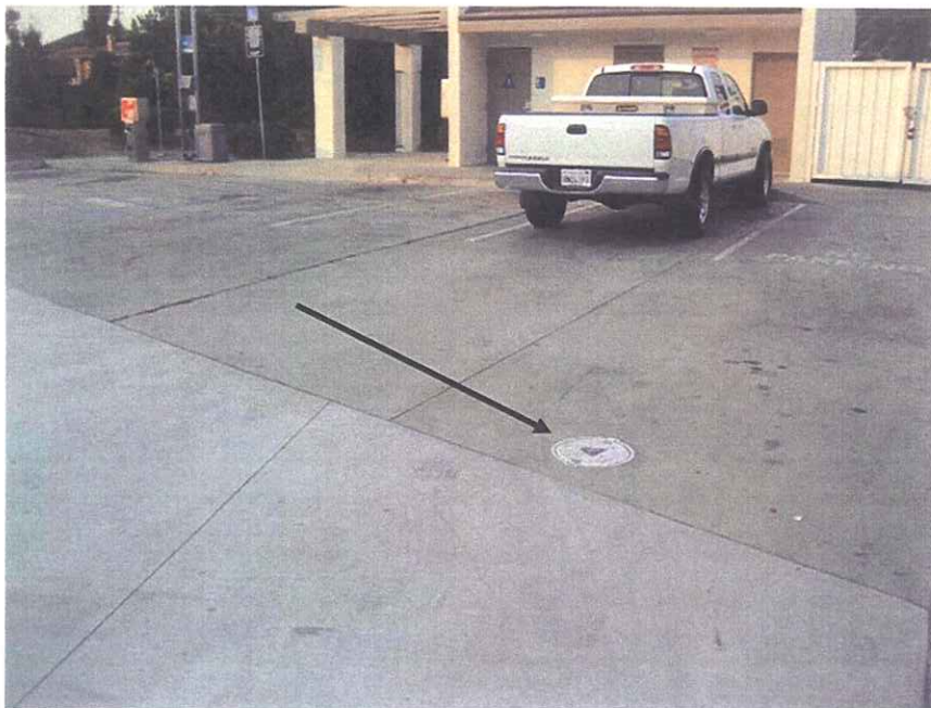
#12 The only groundwater monitoring well located at 5221 Palo Comado Canyon Road. This monitoring well will not be affected by the proposed project.
