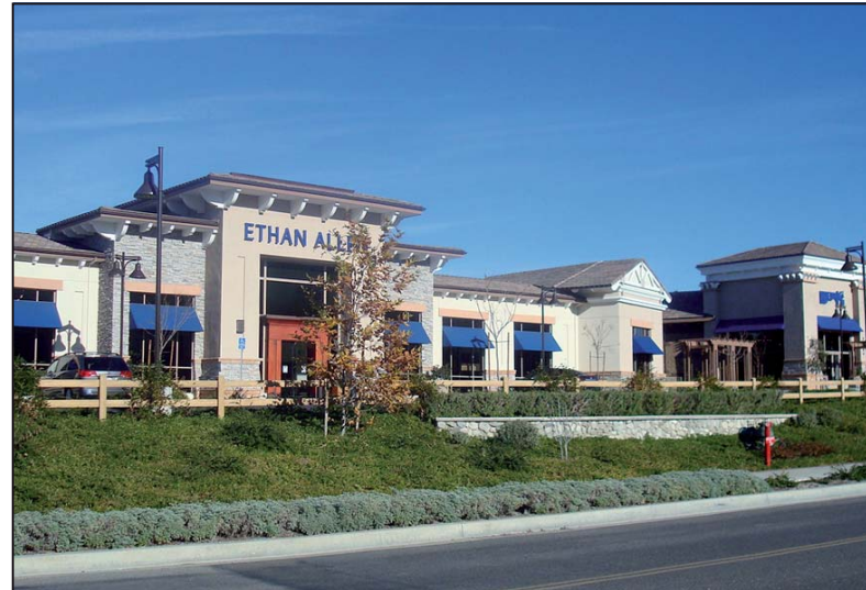
Photo 4 - View of commercial developments east of project site on Canwood Street.
