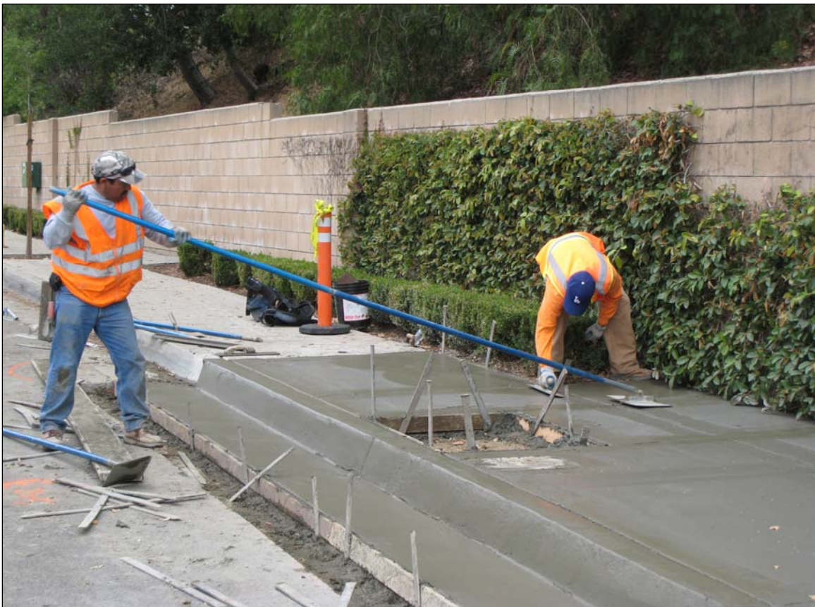
Sidewalk Replacement on Kanan Road
