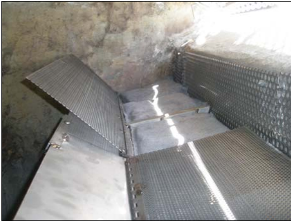
Catch Basin Grates located at Rainbow View Drive
