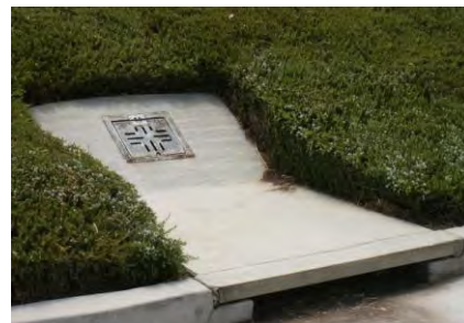
Stormwater drain on Agoura Road and Laura La Plante Drive
