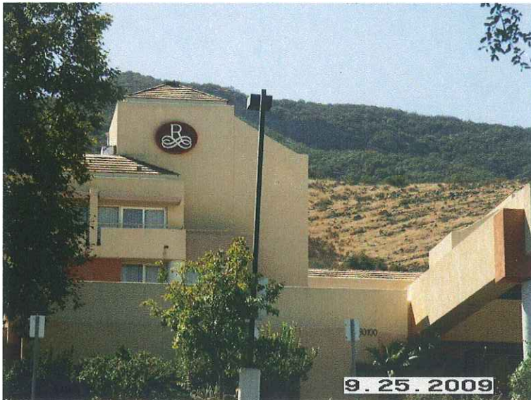
WTF to Right of Renaissance Hotel Sign, Fully Enclosed in Building
