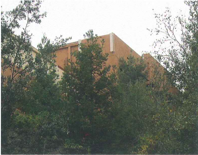
White Panels Side Mounted on Agoura Town Center Building Wall
